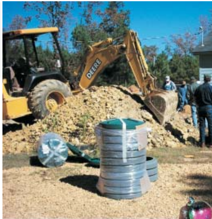
Environmental Supervisor, Wade Bobo holds down the shovel, while several local contractors install the Zabel recirculation device.
