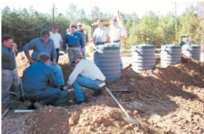
Environmental Supervisor, Wade Bobo holds down the shovel, while several local contractors install the Zabel recirculation device.
