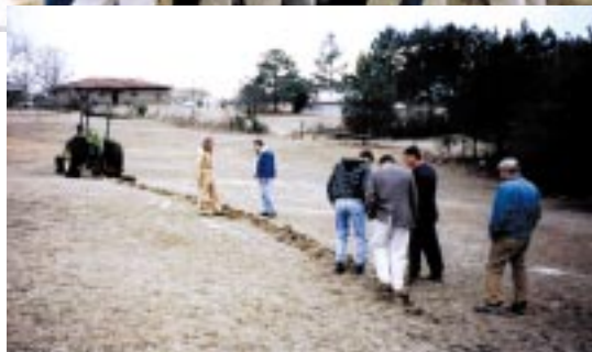
Installing Drip Line with a cut-in blade, very little soil disturbance.
