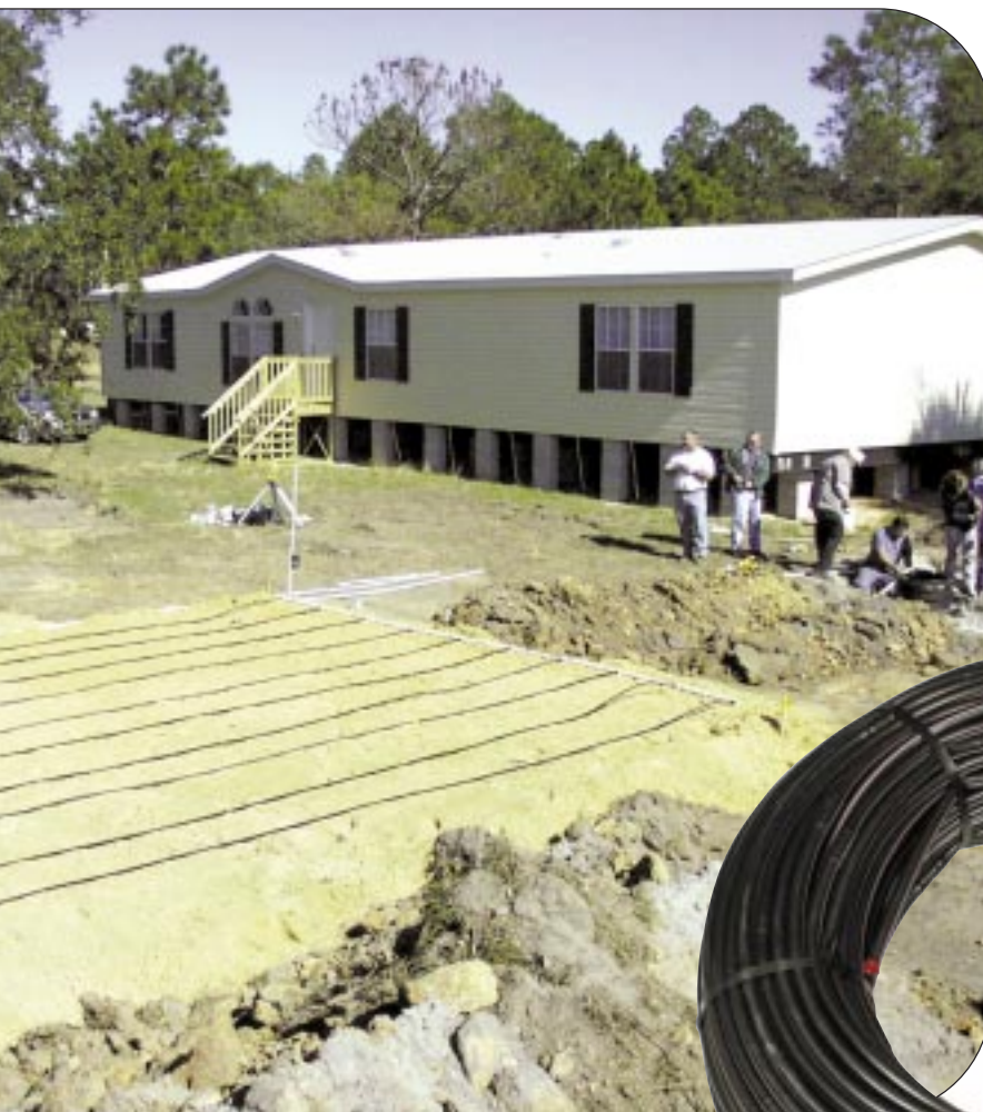
Installation at the Florida Training Center. System Includes: Two tanks to a 10 module AeroCell ATS, then to a dripline bed.
