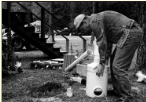
Bill Rawlins assembling the A-300 with reducer
